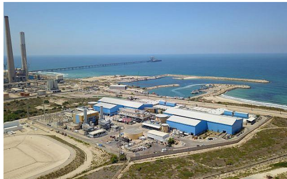
The Ashkelon SWRO desalination facility (IDE) produces 13% of Israel's domestic consumer demand: 100 million m 3 /a, for $0.52/m 3
